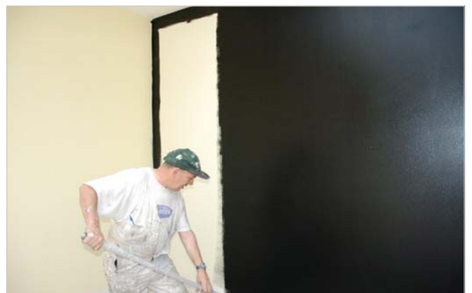
6) Shielding paint is applied.
