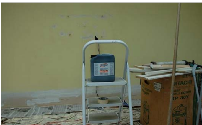
5) Shielding paint about to be applied.
