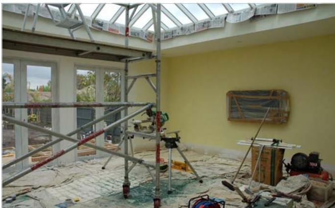
3) Room being prepared for shielding paint application.
